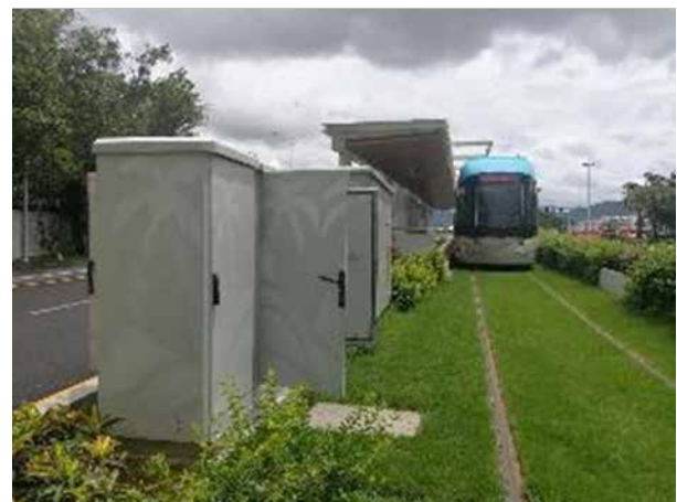
Field Installation, Sanya City, China
